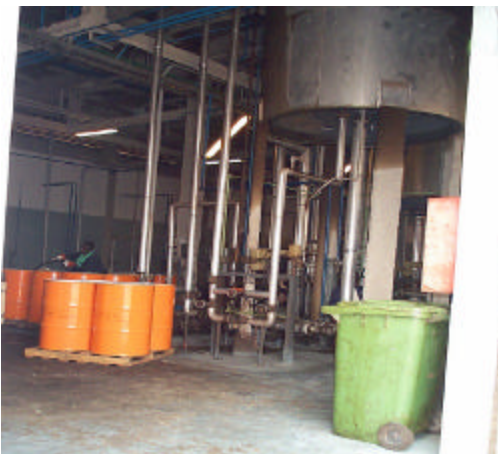
Filling steel drums with lube oil
